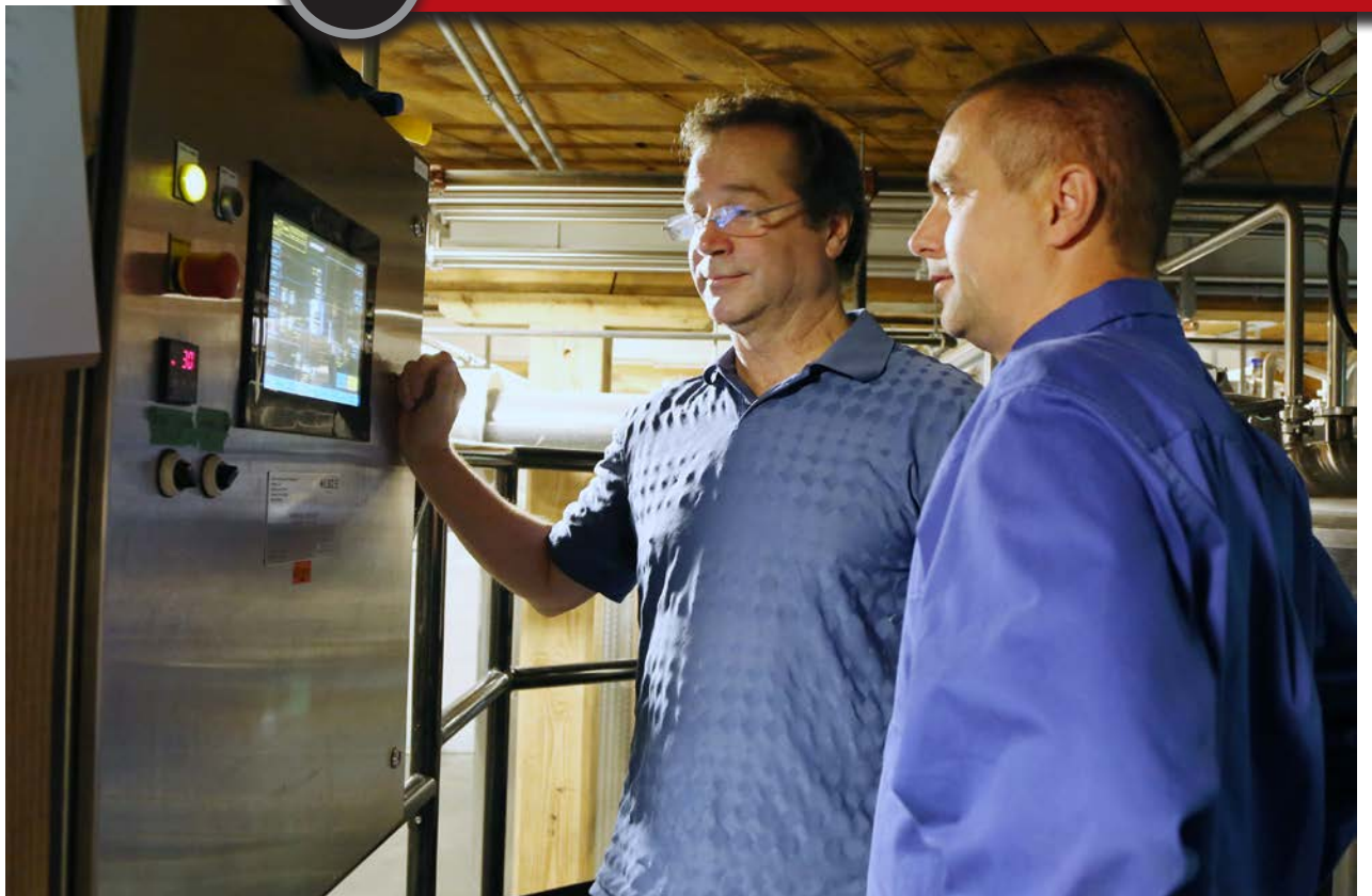
Spring Mill's vice-president of operations Doan Bellman (left) and Jeremy Meyer, territory account manager for central Canada with Omron Automation Americas, taking a look at live equipment status reports displayed in real time on the Omron touchscreen HMI (human-machine interface) terminal embedded into the plant's main control panel.
